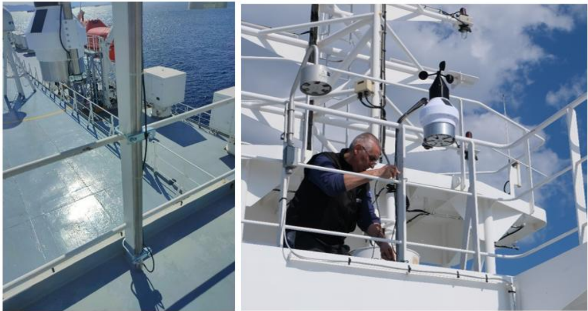
Figure 7.13 Installation of EFOS system
