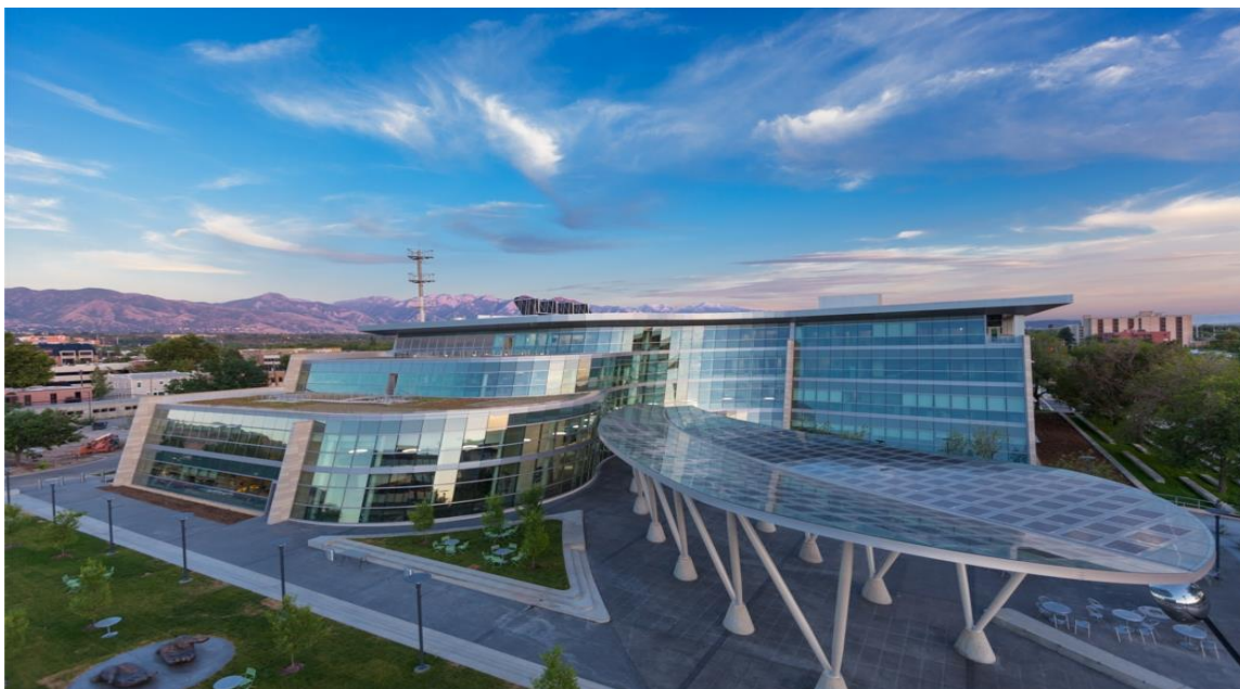
Σχήμα 3.2. The Salt Lake City Public Safety Building. (“New Public Safety Building in Salt Lake City a Model of Resilience – Resilient Design Institute” n.d.)
