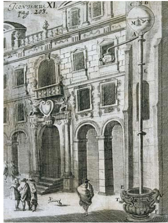
Figure 8.2: Demonstration of void's formation at a street in Rome
