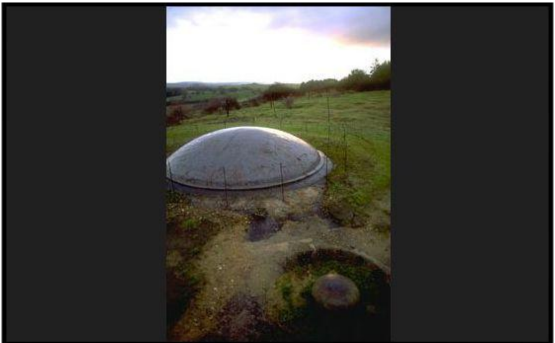
More than 100 retractable machine gun turrets ran the length of the Maginot Line. Photo Credit: Corbis
