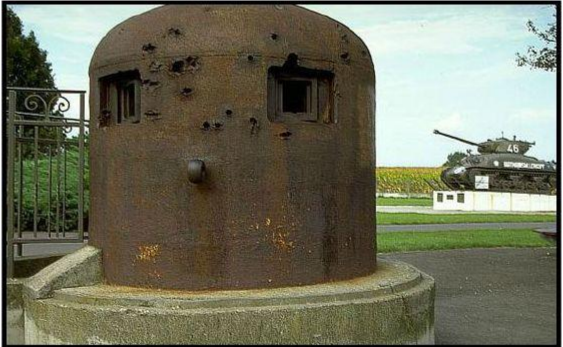
Bell shaped "cloches" made of alloy steel were designed to provide protection for French soldiers at nearly every portion of the Maginot Line. Photo Credit: Corbis
