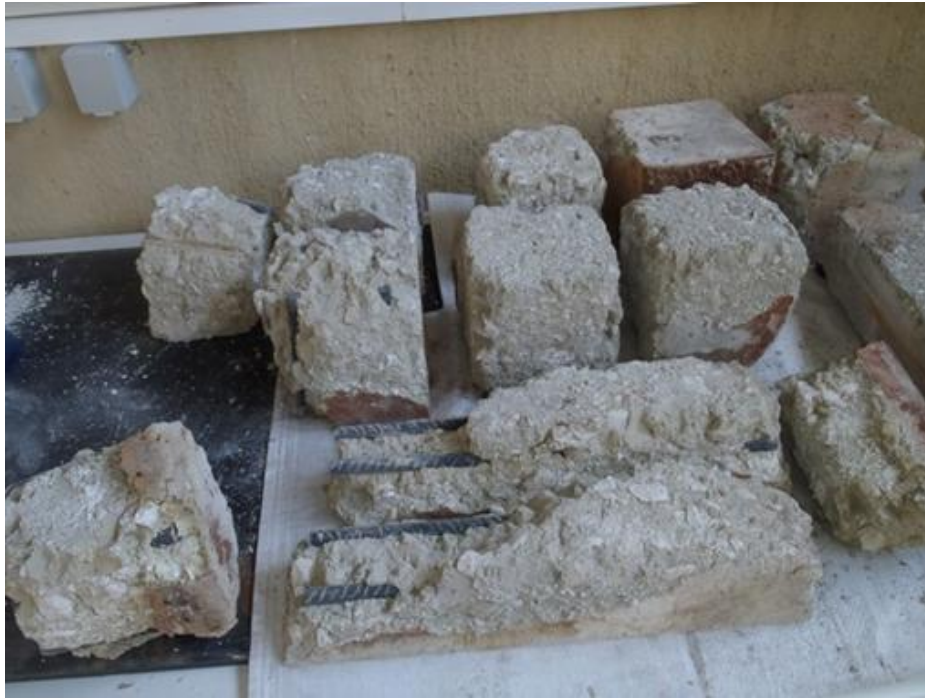
Figure 7. 1 Damaged reinforced concrete specimens after fire exposure.
